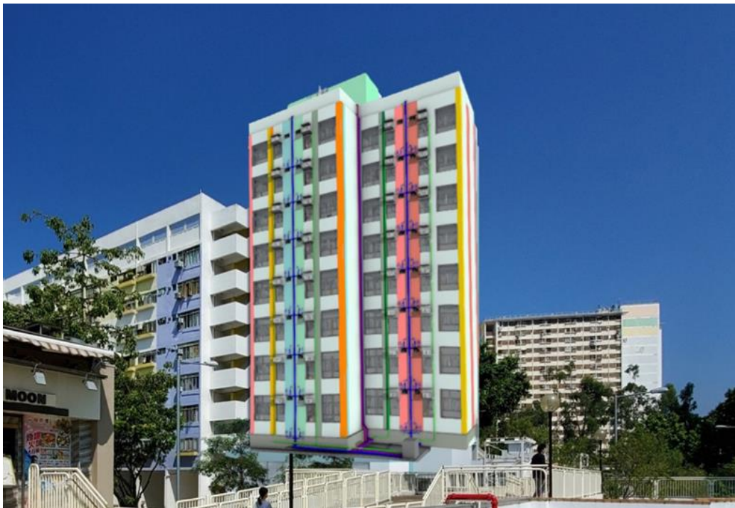
Chevalier Group's first green loan proceeds will be used to construct the Hong Kong Housing Society's first environmentally friendly modular integrated construction ("MiC") elderly housing project - Chung Yuet Lau in Jat Min Chuen in Sha Tin. (This is an artist's impression)
