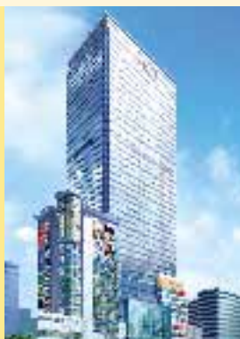
Millennium City 5 intelligent office tower at Kwun Tong – most BEA back office operations in Hong Kong will move in to the new tower by mid-2005.
